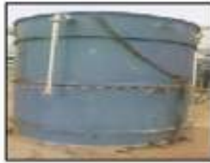
Chemanol Acid Water Tank
