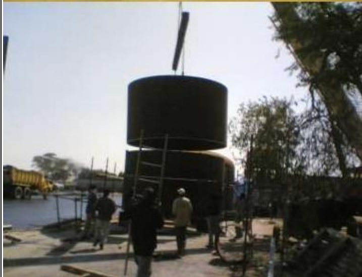
Fabrication of 120 ton Suffer Converter Vessel through INMA Steel Industry for ARAMCO – Khursaniyah Project
